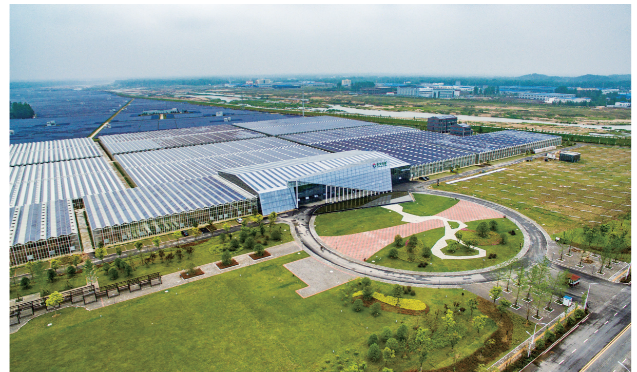
Jinzhai Agricultural-PV Complementary Solar Farm 金寨農光互補電站
