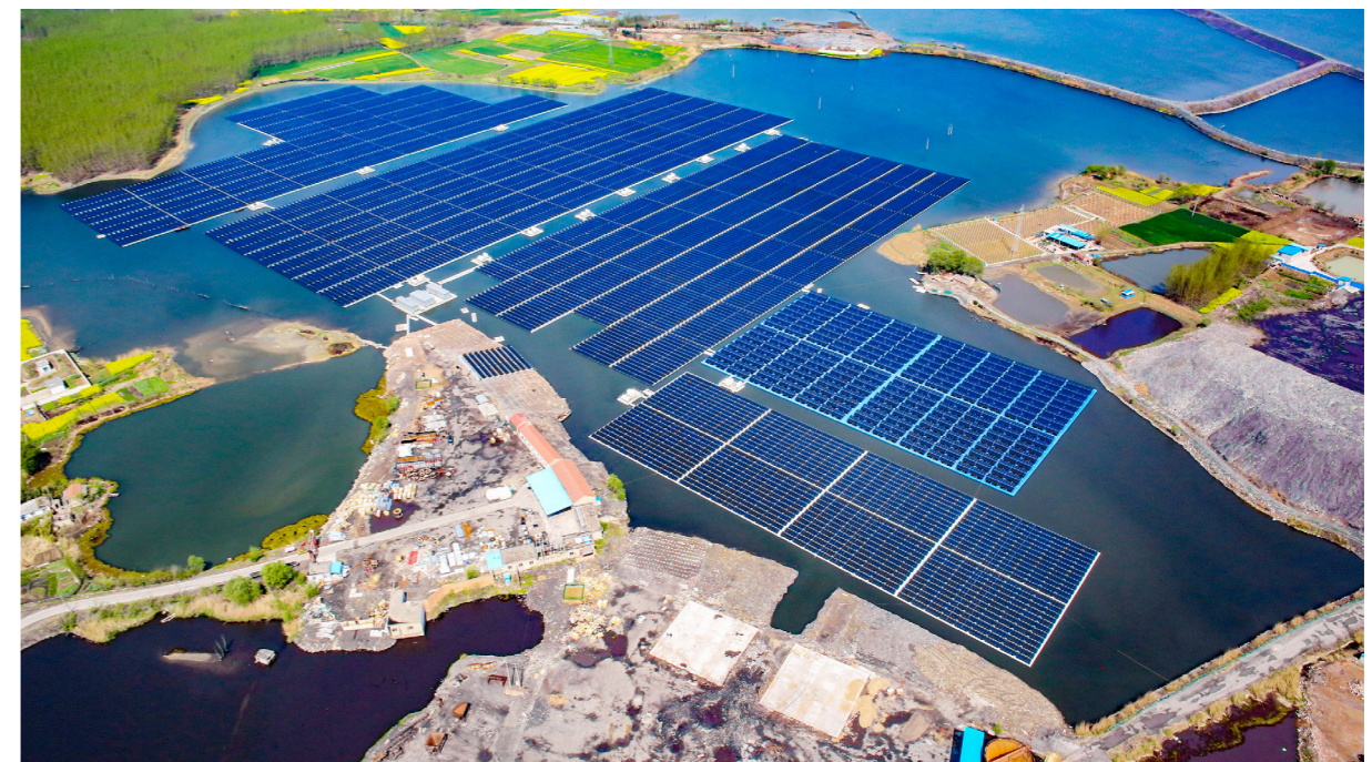
Huainan Solar Farm, with an approved grid-connected capacity of 20MW 淮南電站，核准併網容量20MW
